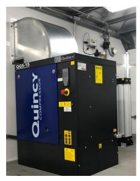
**FEATURES:** Lab & instrument quality air provided by high quality, quiet screw compressors; refrigerated and/or heatless modular desiccant dryer with microprocessor control; particle filter, carbon adsorption filter and all stainless-steel pipe; and tubing; receiver sized to optimize space and to minimize short-cycling.
